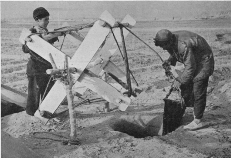
Fig. 2. Excavation of a qanat in Iran (Photography by Cressey, 1958.)
