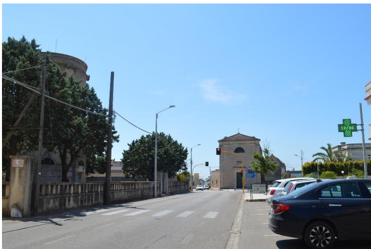
Figure 5 – Square near a tank along Apulian Aqueduct cycle path (Author's elaboration)
